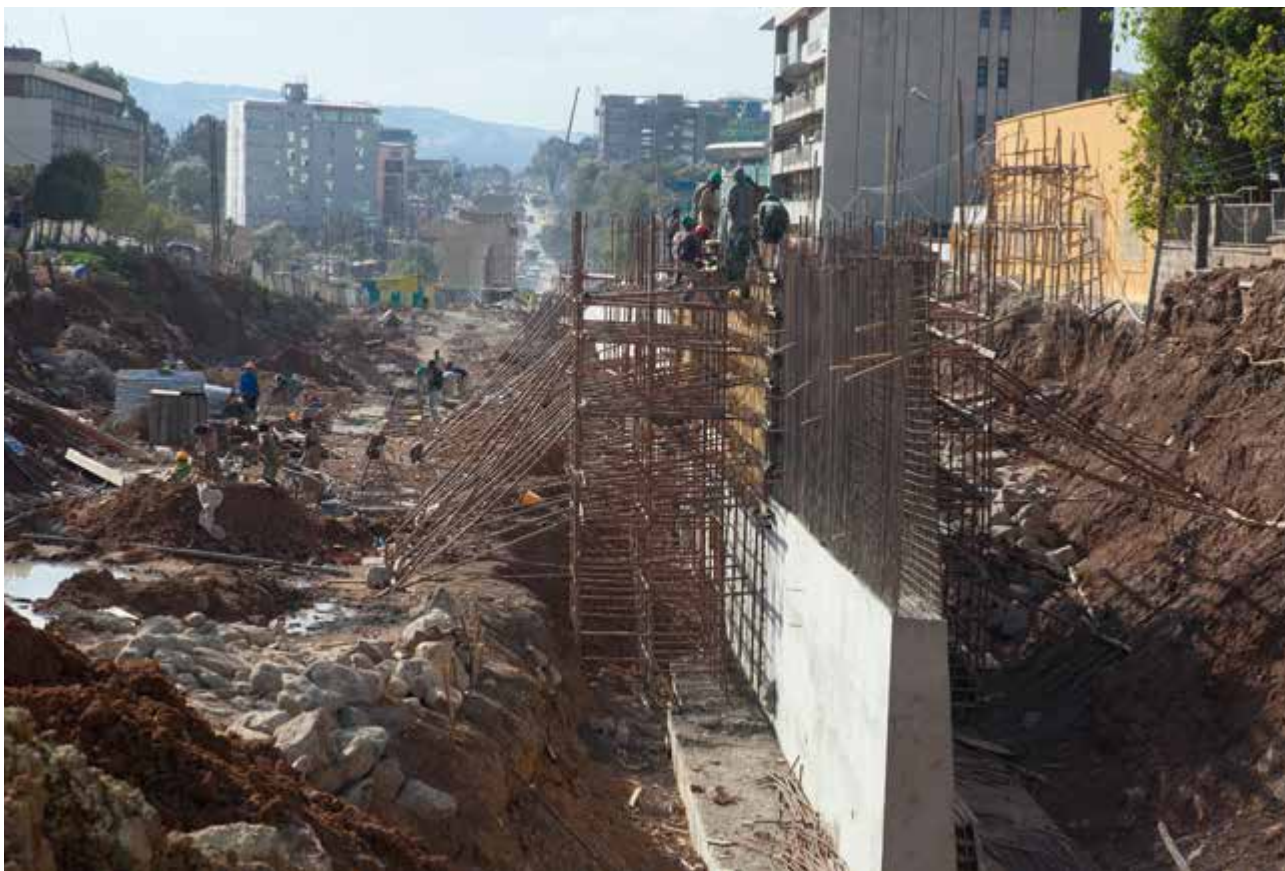
Construction in Addis Ababa, Ethiopia © Shutterstock
