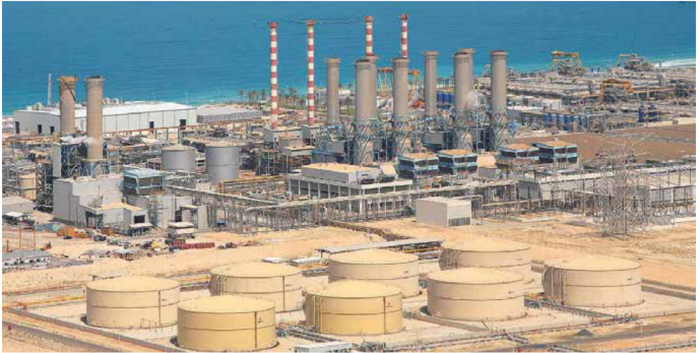
Desalination plant in Dubai, United Arab Emirates © Shao Weiwei-Shutterstock.
