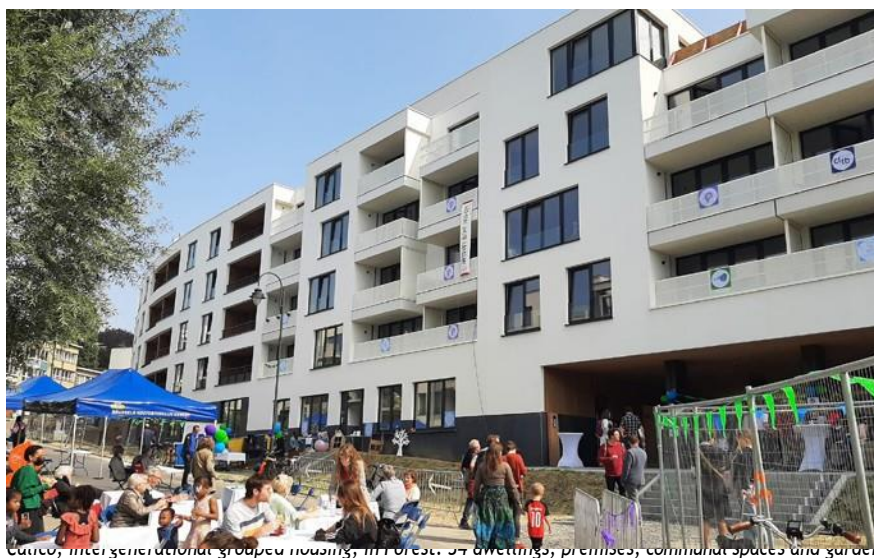
Calico, intergenerational grouped housing, in Forest. 37 dwellings, premises, communal spaces and garden.
