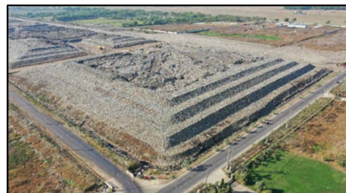
Fig. 17 Landfill site improvement using the Fukuoka Method (in Myanmar)
