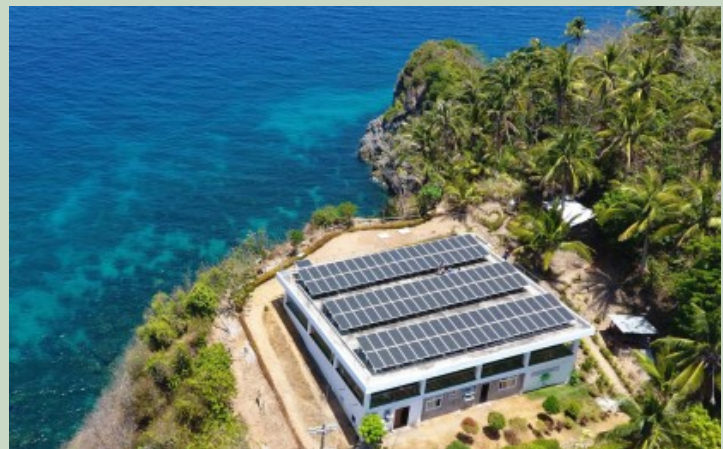
Solar panels installed in local government buildings in Samar as part of wider initiative to foster energy independence amid frequent power interruptions affecting the entire Samar Island Photo from Philippine News Agency, October 21, 2024
