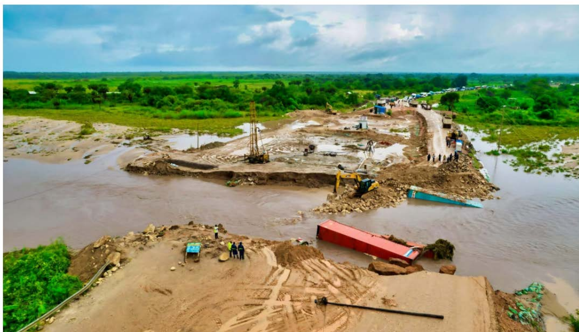
Figure 48: Effects of disasters on road infrastructure, Lindi-Dar es Salaam highway
